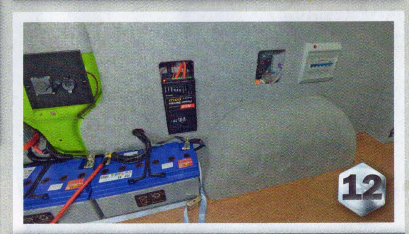
12 A thin sheet of plywood was cut around the charging system and trimmed with Veltrim to finish off. This will all be hidden inside cabinets in time. The vehicle was then started up and all the headlights switched on (to trigger the alternator to start charging). The LED switched from 'solar' to 'alternator' to indicate the power source had changed. Finally, the system was plugged into the mains and the 240V AC LED illuminated. Success!
