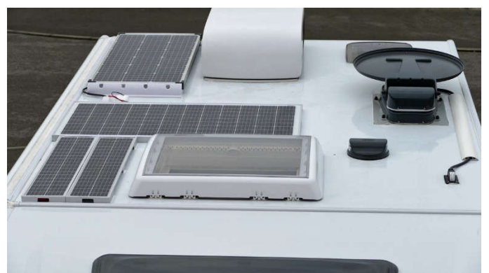
The finished job with 255 Watts of solar capacity.
